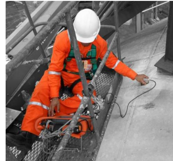
Non-destructive testing (NDT) inspection
